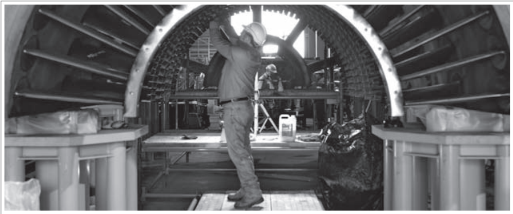
Image (left) Turbine blades were individually cleaned and checked for wear and tear during the Swanbank E overhaul.
